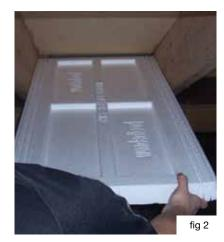
wunderfloor being installed between joists with a snug fit and panel top side must be up tight to the underside of the floor.
