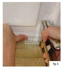
wunderfloor is being further supported by special fitting brackets stapled into place. Other fixing methods can be used.
